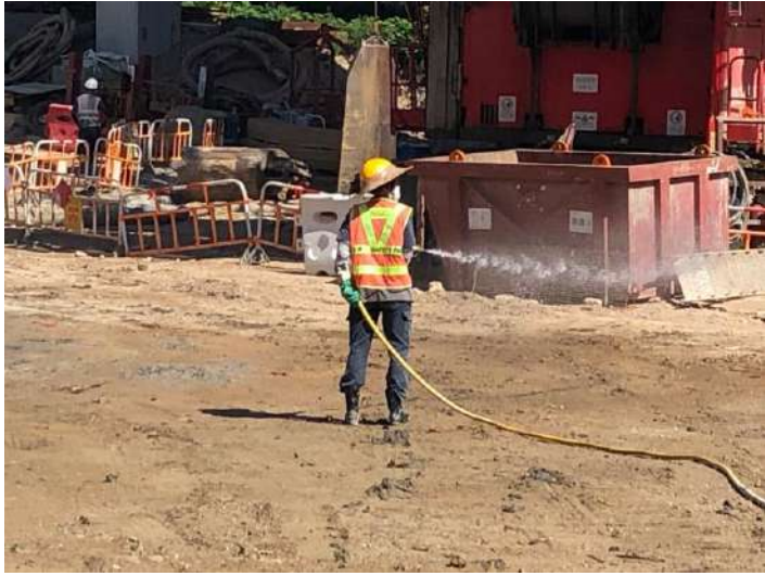
Figure A1 Water spraying
